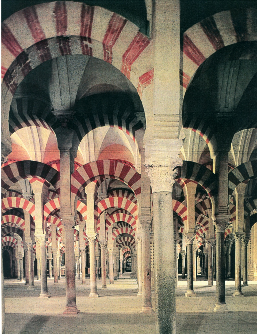
The nave of the Great Mosque of Cordova (begun in 785 by Abd al-Rahman I) with its veritable forest of columns supporting double horseshoe arches of red brick and white stone.
